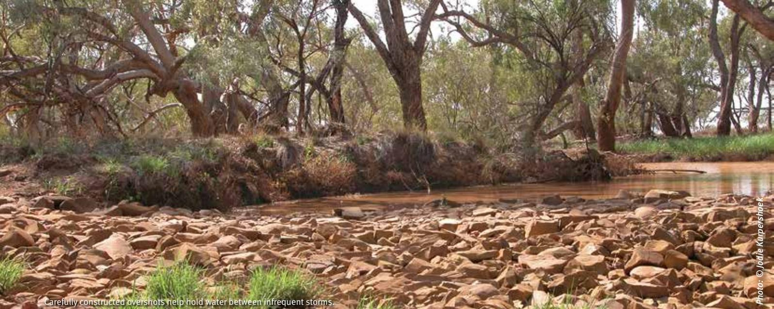
Carefully constructed overshoots help hold water between infrequent storms.
